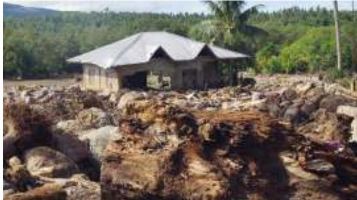
Damage of TS Urduja in Biliran
