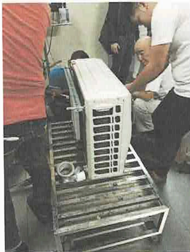
Figure 3. Installation of HB Air-conditioning System
